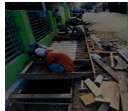
Pelebaran Drainase di Masjid Al-Hakkam Jalur I Furia (260 M')
